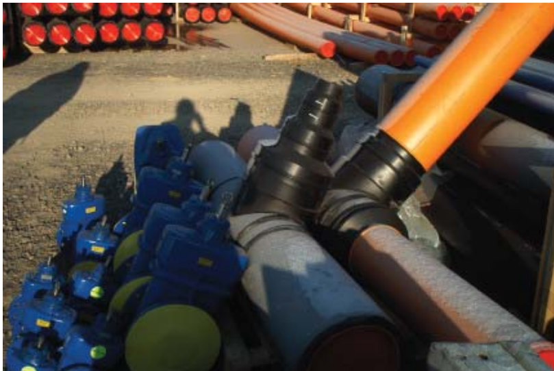
Photo 1: pre-assembled branches for gas pipes and fire mains
