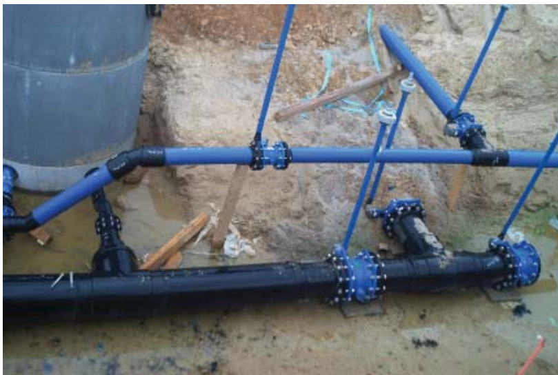
Photo 9: Fittings being fixed in the fire main and drinking water pipe
